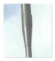
The height of all mmW concealment modules (the Optional Millimeter-Wave Top-Mounting Zone) must not exceed any height that would extend any top-mounted antenna enclosure to a height more than nine feet (9') above the original pole height.
